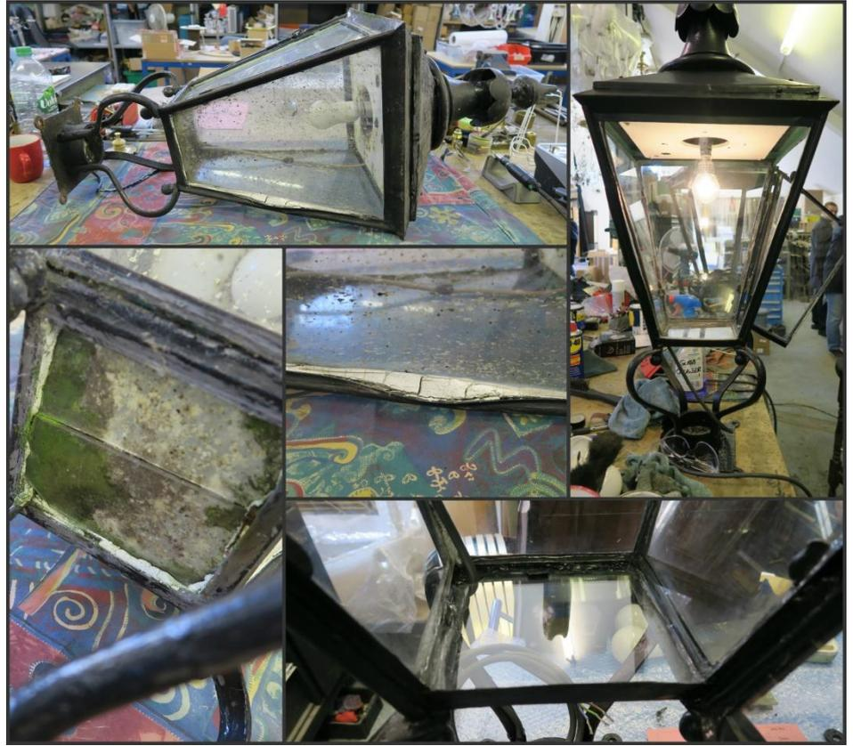
rust was removed, a fresh layer of white waterproof paint was added to the inside. The pair were then rewired with thick waterproof electrical cable and the original / replacement glass panes sealed in to the frame, with sealant that would not expand as it had done previously and damaged the metalwork. The lanterns were finished with one of our dimmable 7w GLS bulbs which should give of plenty of light during the dark winter nights!
